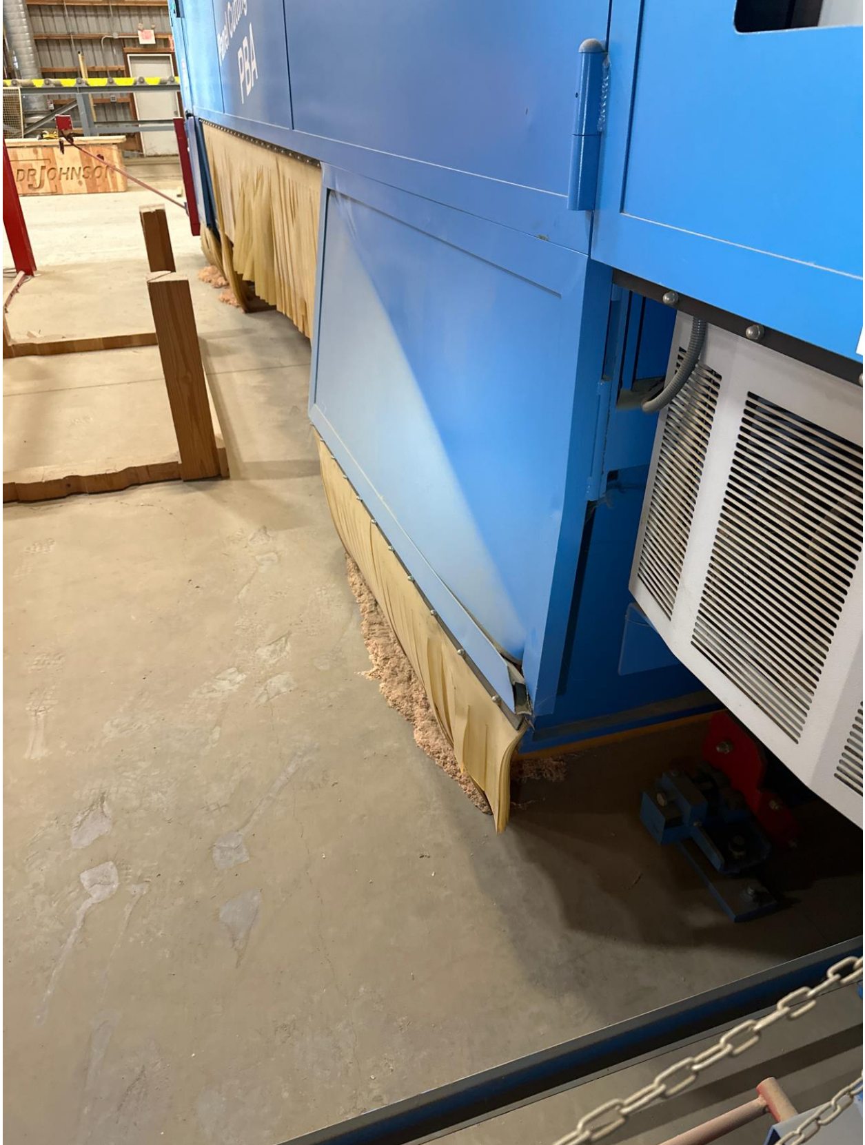
The panel right next to the right hand access door is also bent
